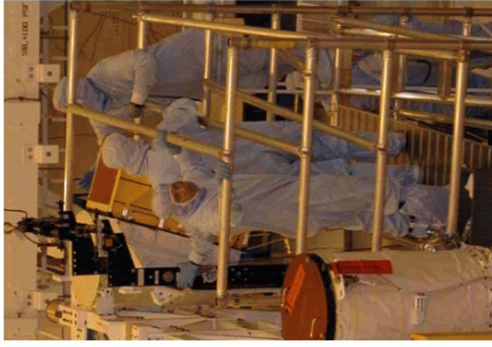
PSRD Lift for GBA Installation
