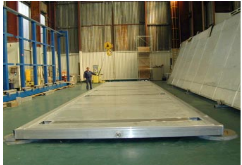
2nd half Module Construction
